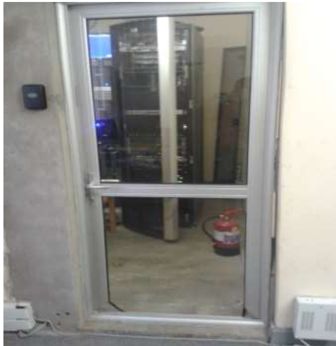
Fig 3: Showing before the installation of Fire suppression door and Biometric System
